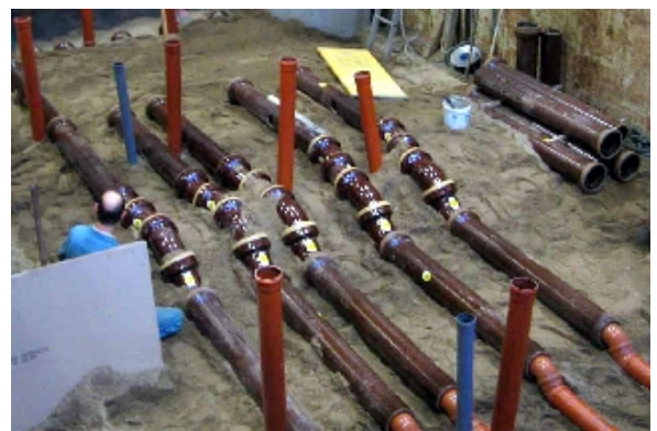
Construction of a sewer
